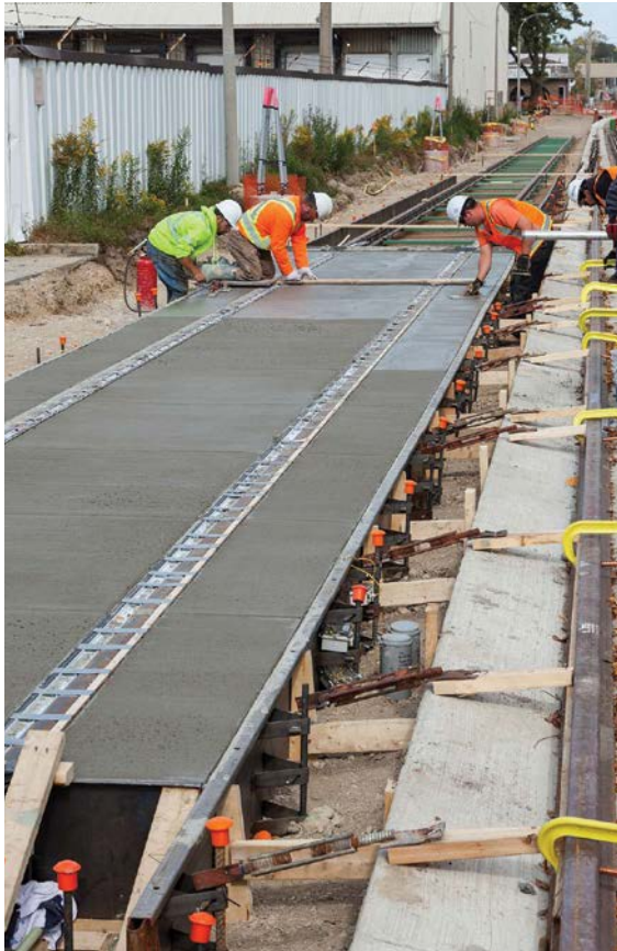
Light rail transit construction, Region of Waterloo
